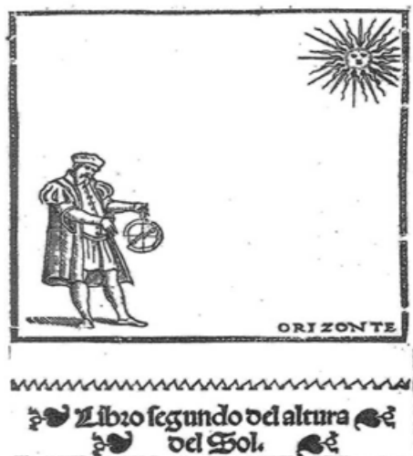
Plate 100: Illustration of Pedro de Medina's Regimiento de Navegación , 1563, with instructions for the proper measurement of the height of the sun with an astrolabe.
