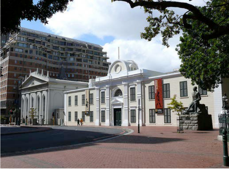
Plate 83. The Slave Lodge of the VOC in Cape Town, South Africa. Built in 1679 to house the slaves brought from Indonesia and the rest of Africa who were working in the gardens of the Company.
