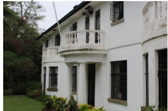
Exterior of the building
