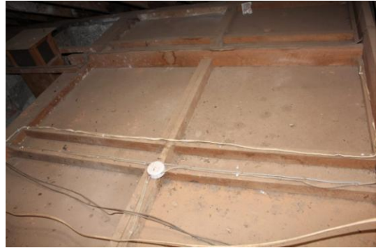
Asbestos ceiling
