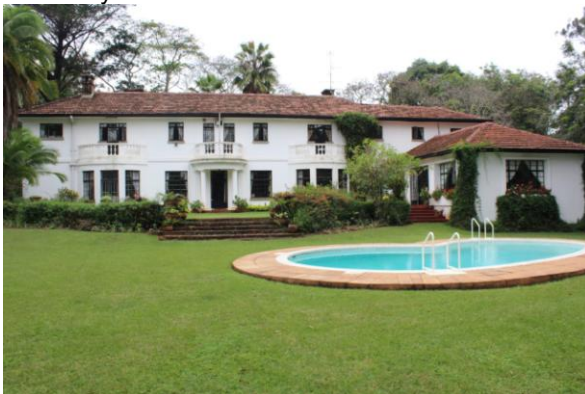
Exterior of the building
