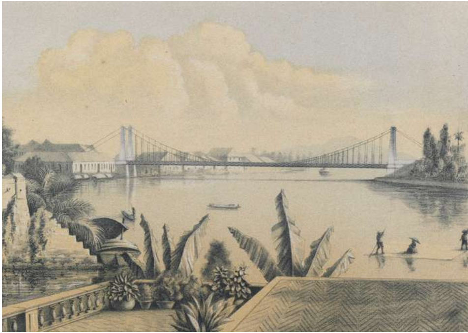
View of the Suspension Bridge, taken from the Escotta. 15 May 1859. Baltasar Giraudier, lithographer. Facsimile reproduction. National Library, Madrid, Spain. ER/2241 (8).
